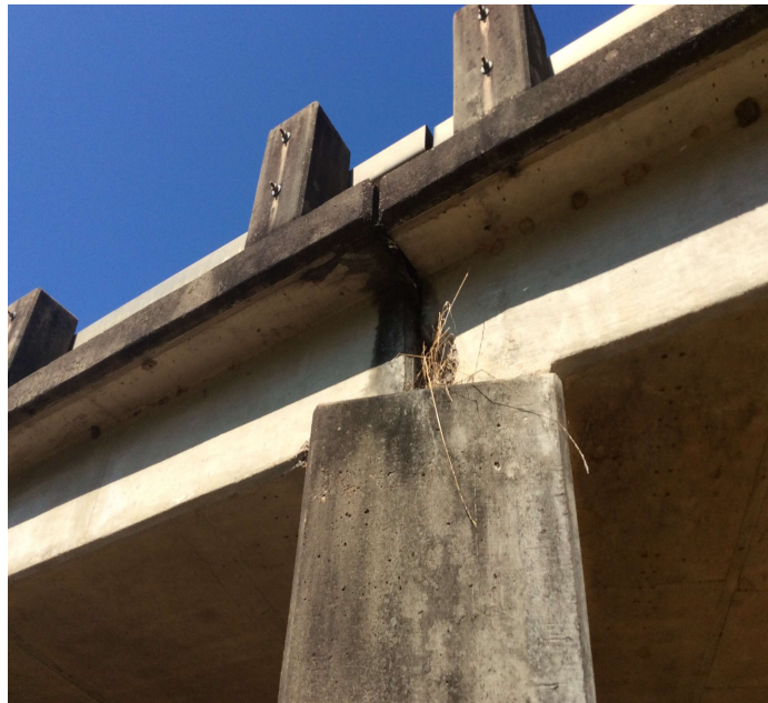
PHOTO 1 Description Bent 3 left side spall in corner of slab
